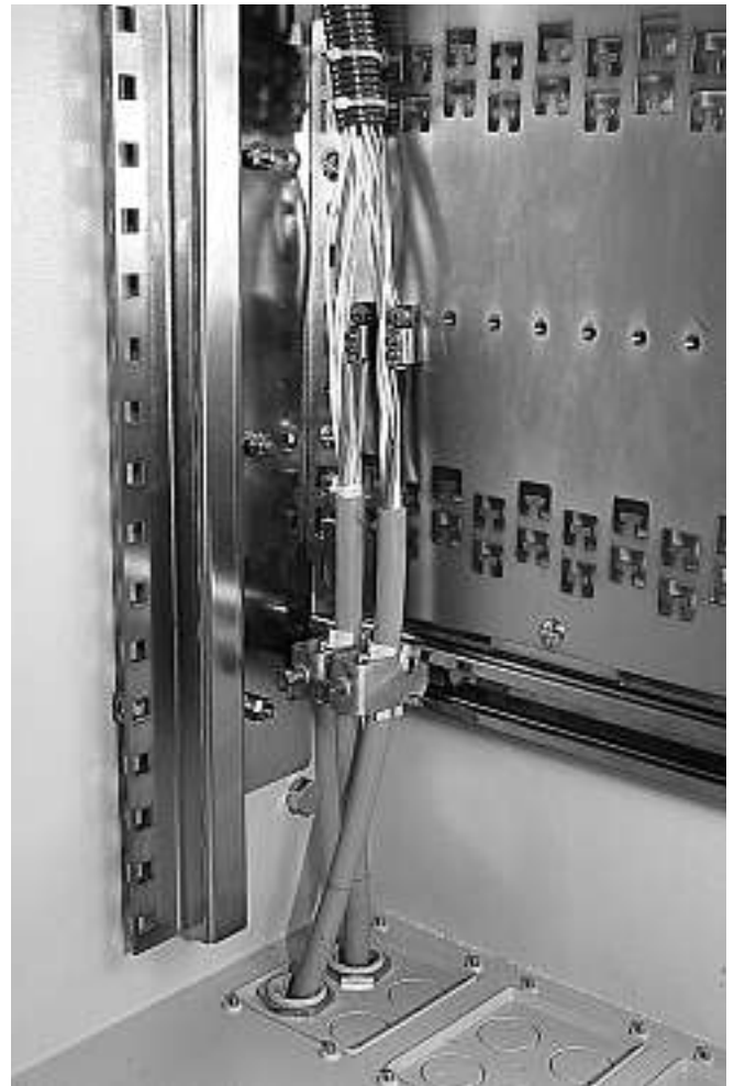
7.6 Using two cable clamps on two cables.
