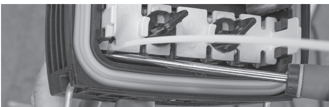
5.4 Use a flat screw driver to push the cable jacket in to the spring. Tighten the trigger as standard practice
