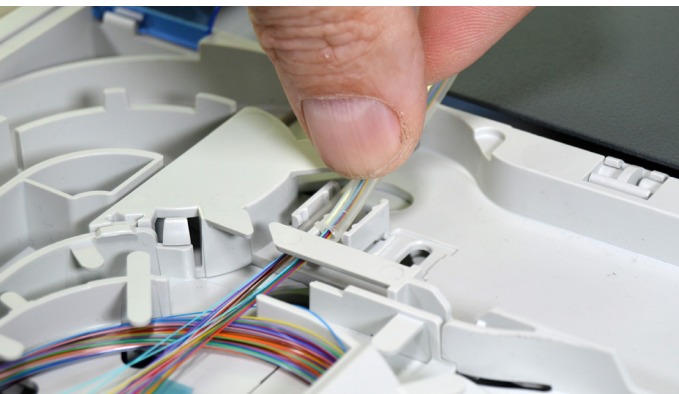
7.2.5. Place the additional tube, if needed.
