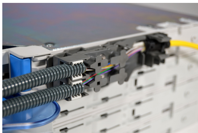
6.4. Slide on the CTU bracket. Fix the flex tubes by pressing the flex tube(s) into the flex tube holders.
