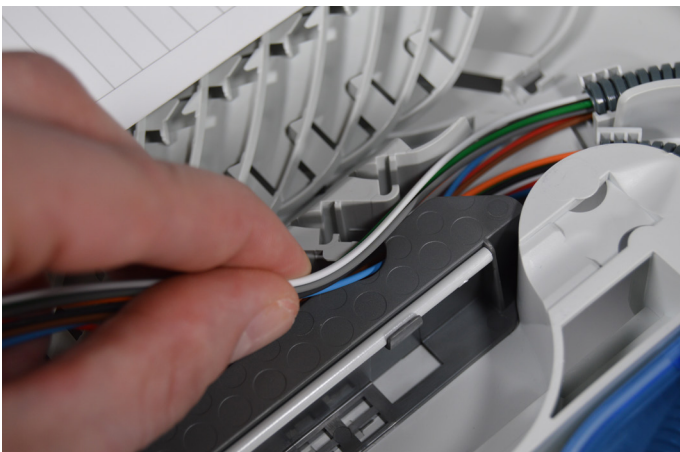
6.8. Route the fibers throughout the groove plate to the dedicated splice trays.
