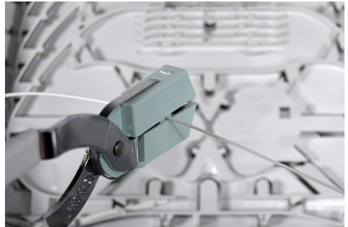
6.10. Strip the 900 \mu\text{m} to 250 \mu\text{m} with a proper tool.
