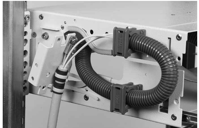
4.2.10 Fasten the flex tube at the bottom tube holder and afterwards at the top. Attach the push tie wraps onto the plate and fasten the strength member connector. Mount the cover on the flex tube holders.
