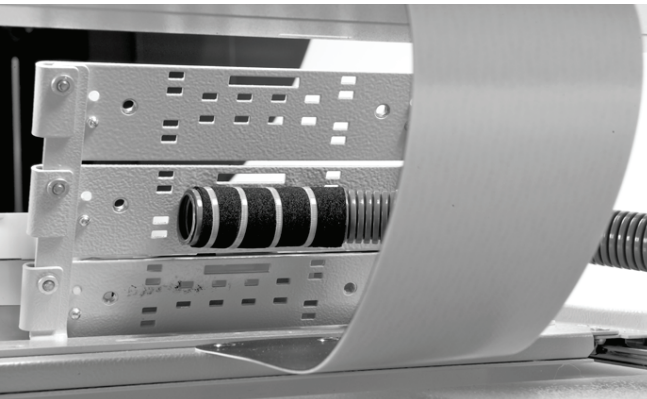
5.2.10 Make sure the flex tube is long enough for the drawer to slide easily in and out. Secure the flex tube using four tie wrap and foam as shown on the pictures.
