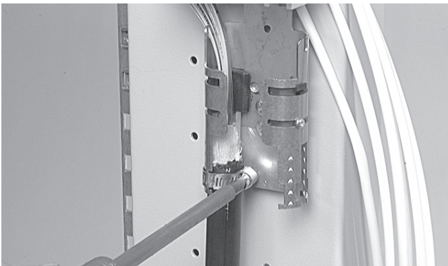
4.1.24 Secure with the cable clamp. Don't squeeze the cable.
