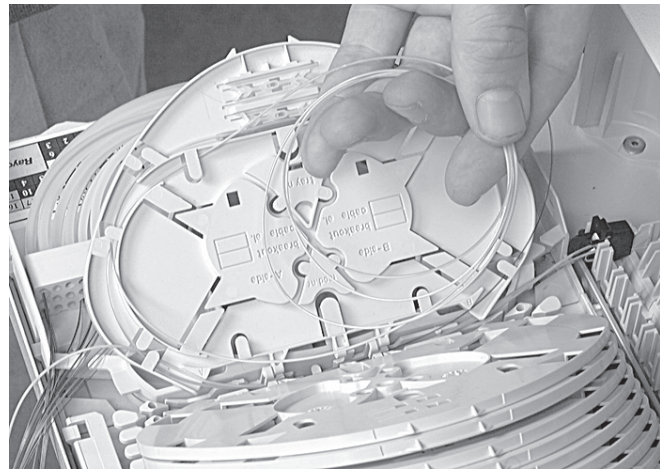
6.1.2 Guide the fibers in the groove plate. Make sure all fibers are positioned under the lips. Splice the fibers and protect the splice. Position the splice in the spliceholder.
