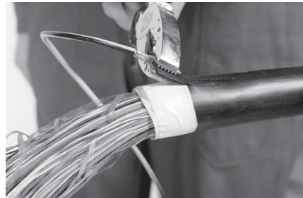
4 Install a shield continuity wire on each cable using a standard pair of pliers.
