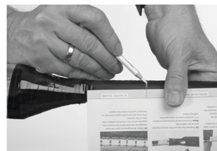
11 Use measuring strip of the corresponding BOKT (at bottom of installation instruction) from the end of liner/canister and mark the bondline length on each cable.
