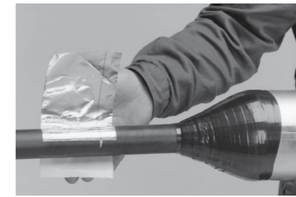
13 Apply the aluminum foil to the cables, positioning the blue line at the mark of the bondlength and smooth the aluminum foil.
