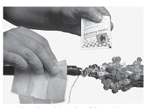
6 Clean the cable jacket of the cables using the delivered cleaning tissue.
