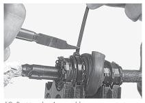
19 Position the 4-out cable separator in between the cables (or plugs), insert in the central part and tighten the tie wraps.
