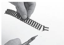
11 Cut the first tape element as shown, but do not cut the element completely off. The partially cut element can be held against the cable and used as an installation aid when wrapping the tape.
