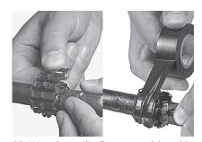
12 Wrap the axial pull tape around the cable using loose lid to keep the strip in place. Use PVC tape to secure. On each cable two axial pull strips with the same length need to be installed on left and right of the marking lines. Remove the partially cut element from both tapes.
