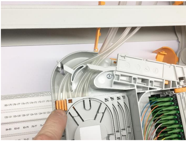
10.5.13 Remove the splice tray cover. Push the tube holders into the splice trays, follow the correct slot for guiding the FOPT tubes.
