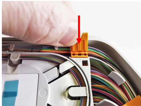
10.7.2 Replace the pigtail for a new one and insert all pigtails back into the 900µ holder and push them down with the 900µ insertion tool.
