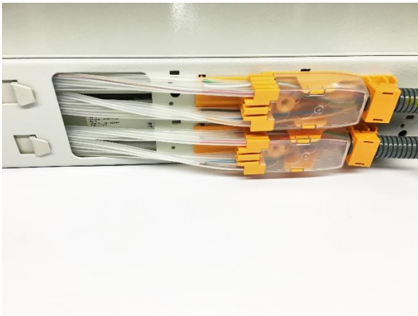
10.5.19 Place the covers on the CTU-L brackets.
