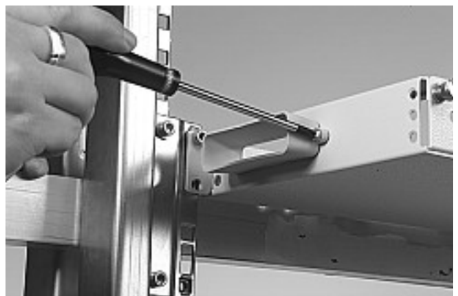
3.1.2 Trumpet is needed where the pigtails enter the shelf. Depending on the rack configuration it is possible to install the trumpet at the left (in case of right version) or at the back side of the shelf.
