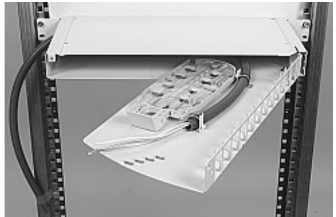
3.4.11 Termination of cable in the rack, entering the shelf from the side, also possible entering at the back. Next step see 3.4.3.
