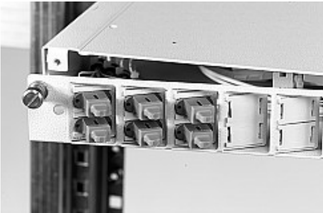
3.2.1 Place the connector-adaptors in the patchpanel. In the picture you also can see the blind stops.
