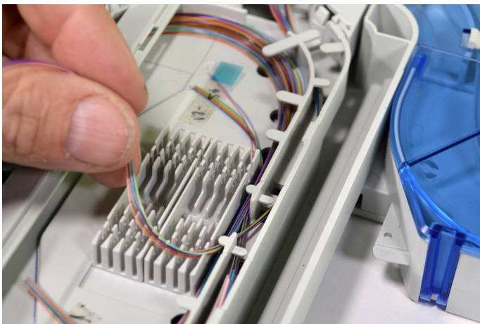
7.2.6. Guide the fibers into the splice island.
