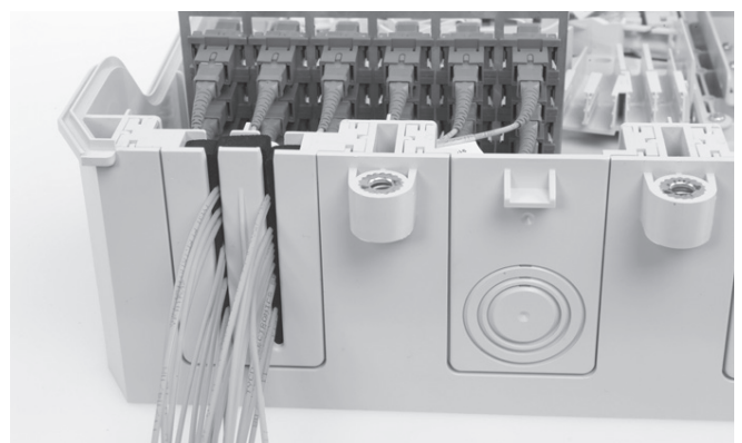
6.2 Install the next 12 patchcords and route these into the second groove of the seal.
