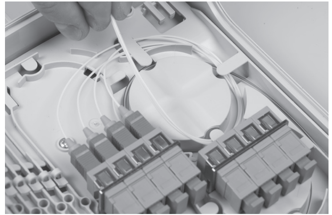
4.4 Connect first four 900µm pigtails.
