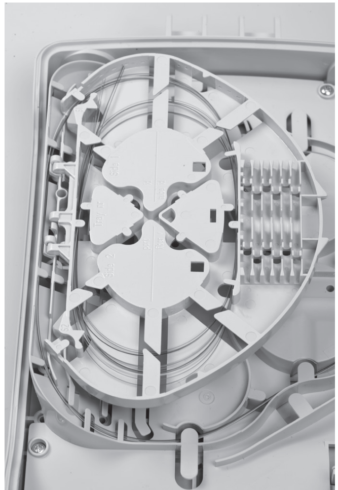
3.12. Route the fibers to be spliced towards to the tray trough the Box as shown.
