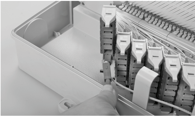
7.1 Slide the patch panel upwards until the first locking position, not further. Connect the pigtail/patch cord into the designated adaptor.
