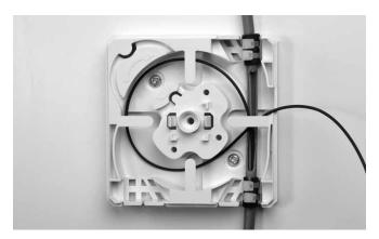
4.3 Routing the fiber in the base tray up to the splice tray.
