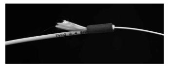
5.1.1 Strip 1 m of the pigtails to 900 micron. Place some Kevlar under the foam, wrap 1 layer of foam around the pigtail at the end of the coating.
