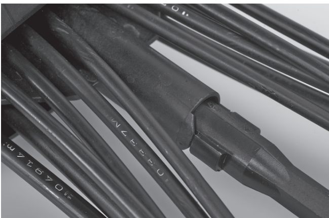
6.7 Tighten the trigger till the wings butt up with the plastic tube.
