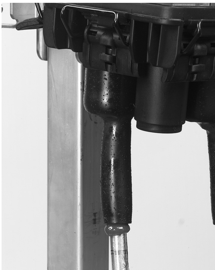
8.2.2.4. Drop cable sleeve installed.
