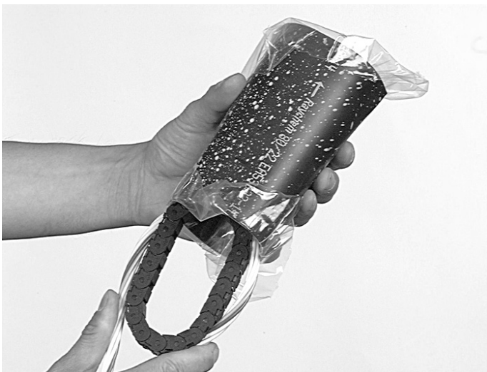
7.2.5.1. Open the oval port; the cutting wire can be used.
