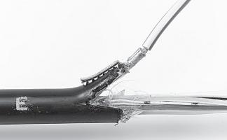
7.1 Install the grounding wire as shown on the picture.
