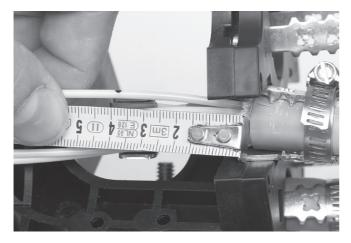
4.4.1 In case of a loop, select the appropriate loose tube and cut in the middle. Strip the loose tube at 40 mm from the jacket.
