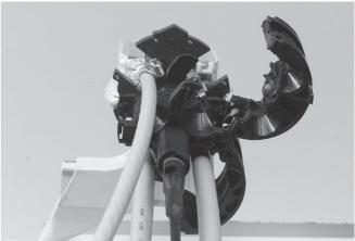
5.2 Position the gel block with the hinge facing the right. Small ports onto main cables, larger ports onto drop cables.
