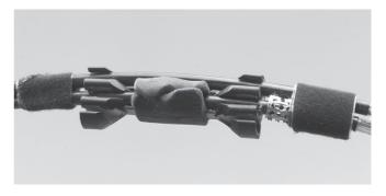
4.3.9 Attach the strength member bracket to the cables. Wrap two complete layers of felt wrap around the cable(s) at the jacket end.
