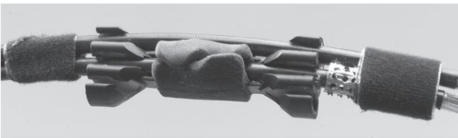
4.2.5 Flip the gel wings together and press to seal around the middle cable.
